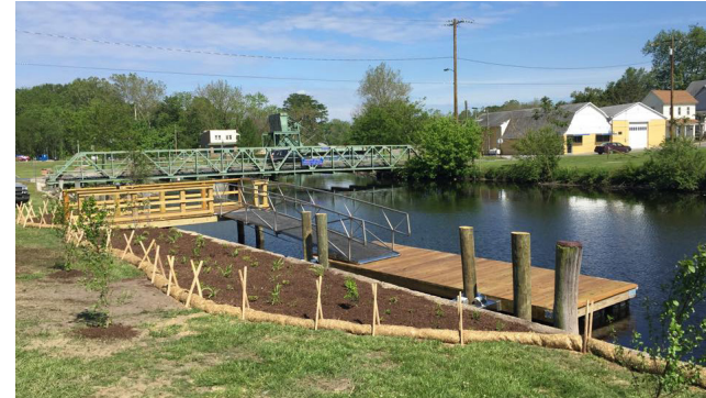
Left, this boat launch was part of The Ramble concept plan. It was built by the Nanticoke Rotary Club. Below, a Habitat family moves into a newly renovated home, thanks to Laurel's Strong Neighborhoods grant.
